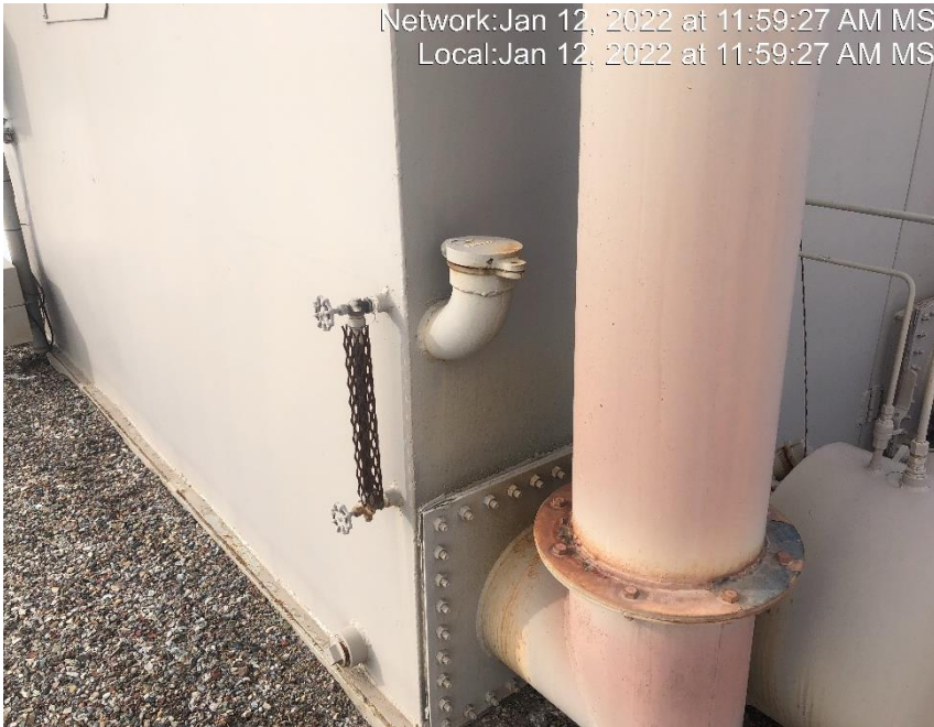
Photo #5661 Sight glass indicates that the storage tank is full of an unknown fluid.
