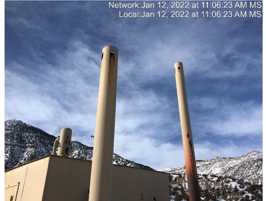
Photo #5653 missing bird protectors.
