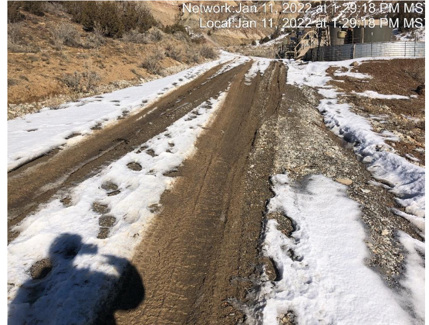
Photo #5650 Insufficient tracking BMP located at entrance to location.
