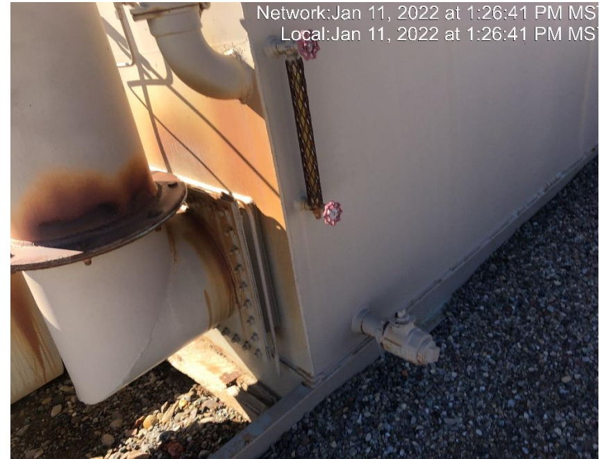
Photo #5648 Sight glass indicates the storage tank is full of an unknown fluid.
