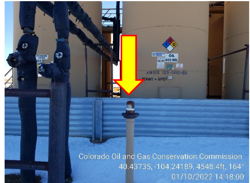
Photo 18 – Unmarked Riser on North Side of Tanks
