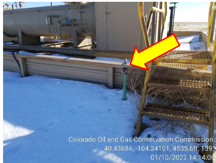
Photo 6 – Unmarked Riser at Separators
