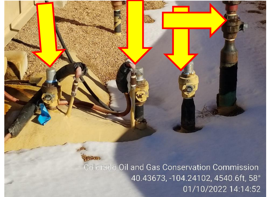
Photo 8 – Unmarked Risers at Separators
