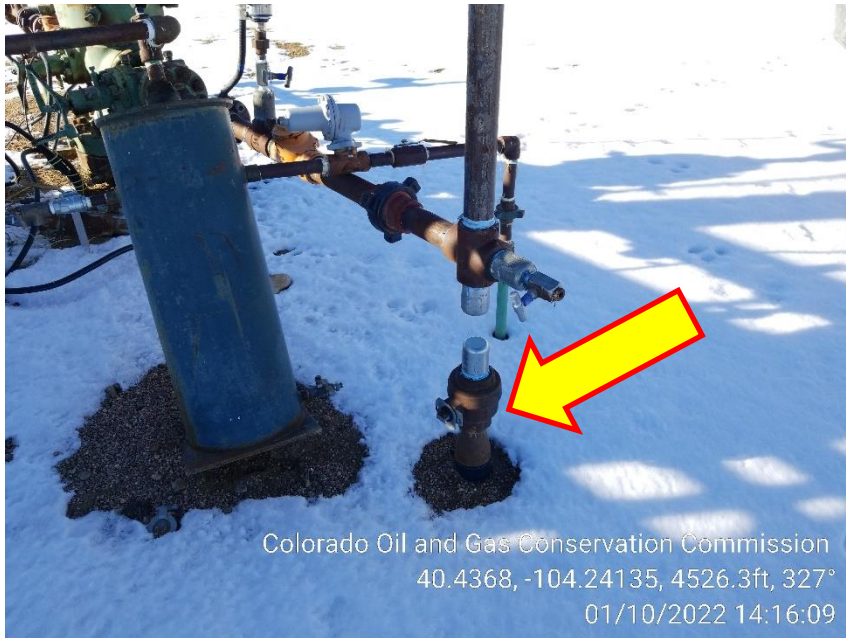
Photo 3 – Unmarked Riser at Wellhead
