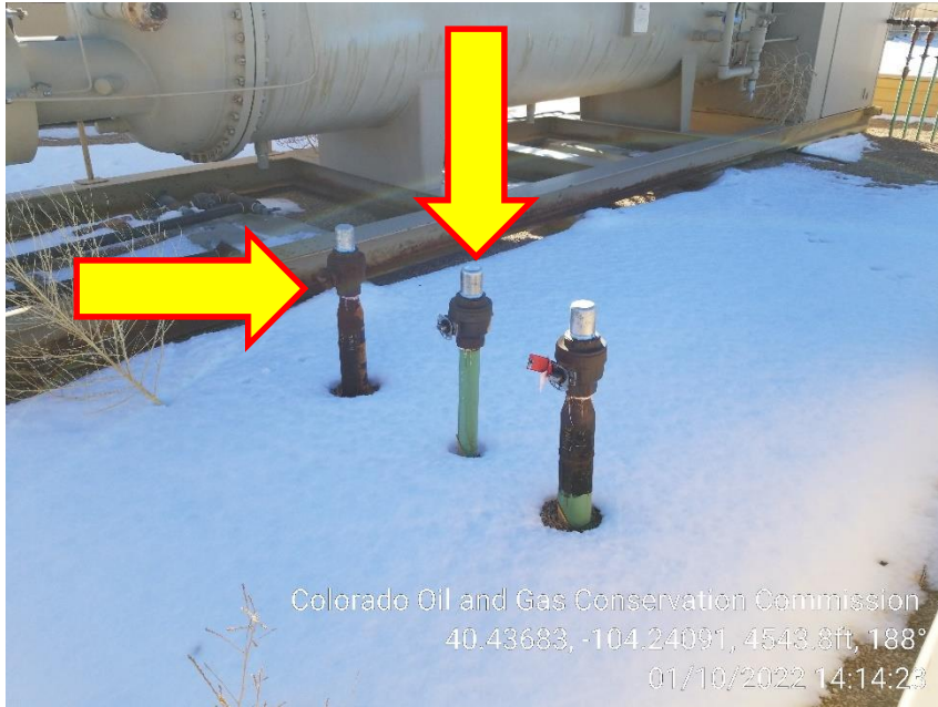
Photo 7 – Unmarked Risers at Separators
