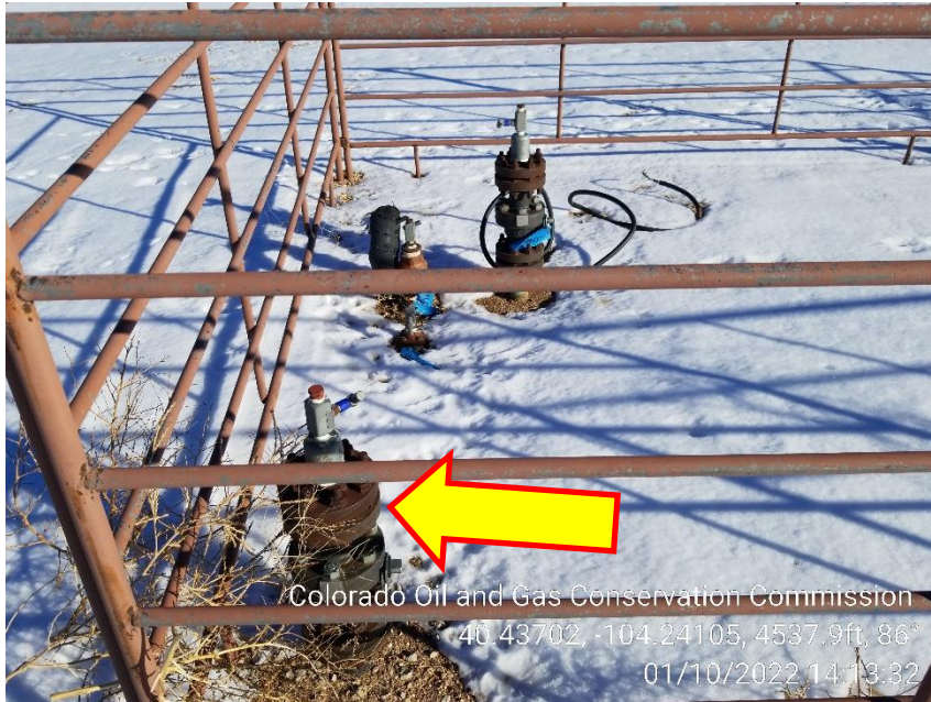
Photo 13 – Unmarked Riser
