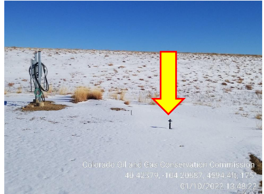
Photo 6 – Unmarked Riser at Pumping Unit
