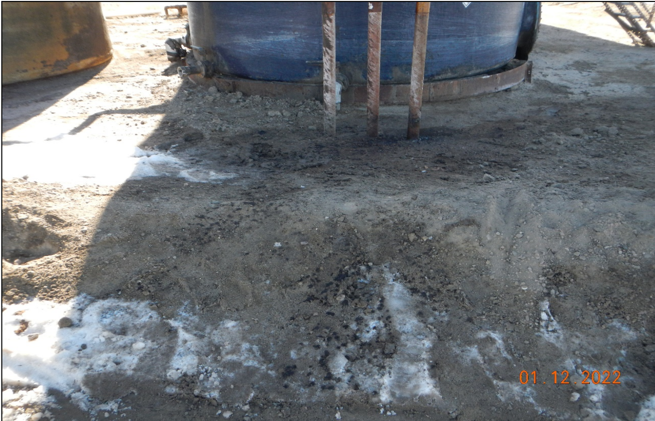
Photo 2. There is oil stained soil from where trucks are loading out the fluids of the tank.
