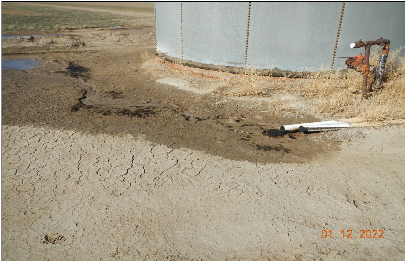
Photo 6. There is E&P waste draining out of this tank overflow pipe.
