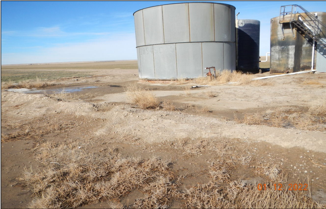
Photo 6. Facing northwest toward the tank battery. The berm around the tanks is not sufficient to contain a spill.
