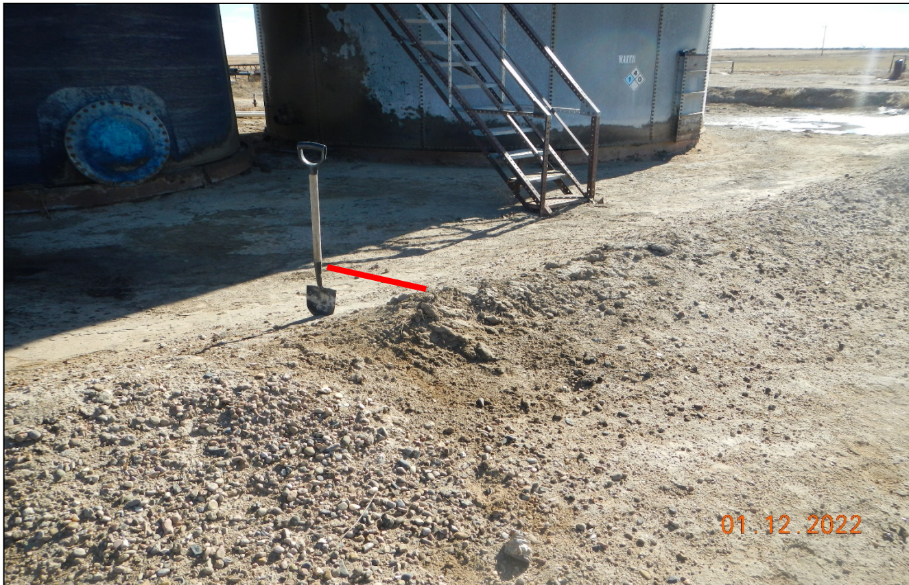
Photo 5. The berm around the tanks is not sufficient to contain a spill. The 3 ft. shovel was placed to show size of the berm which is approximately 12 inches at red line.
