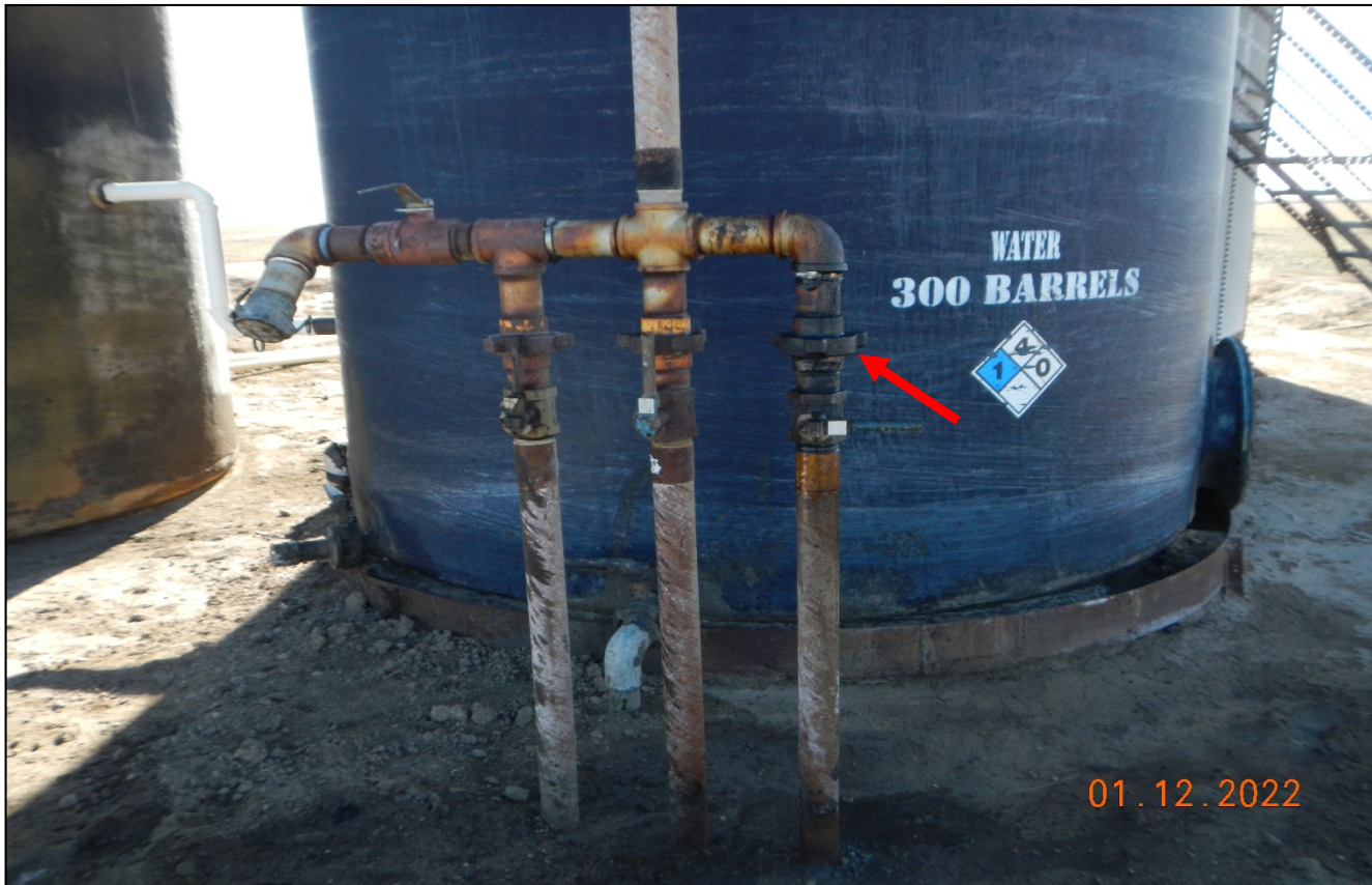
Photo 3. There is water leaking out of the pipe shown at red arrow.
