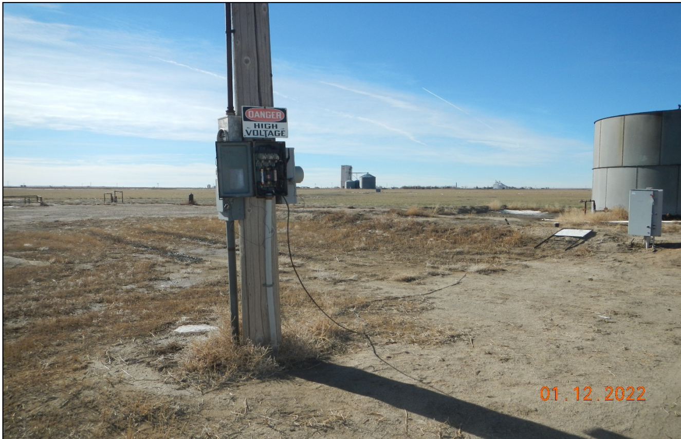
Photo 9. There is an active electric utility that is not secured and protected and is a safety concern. The box needs to be closed and secured and the electric line needs to be protected.
