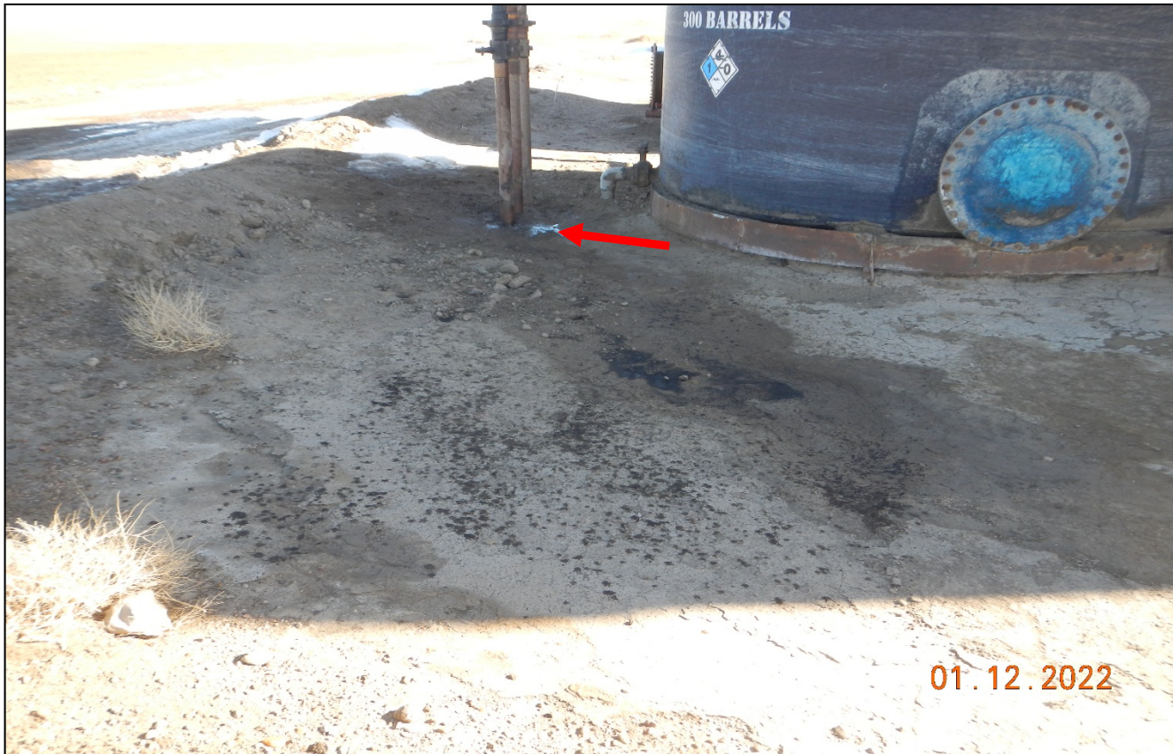
Photo 4. There is oil stained soils and evidence of water leaking out of the pipe shown in previous photo.
