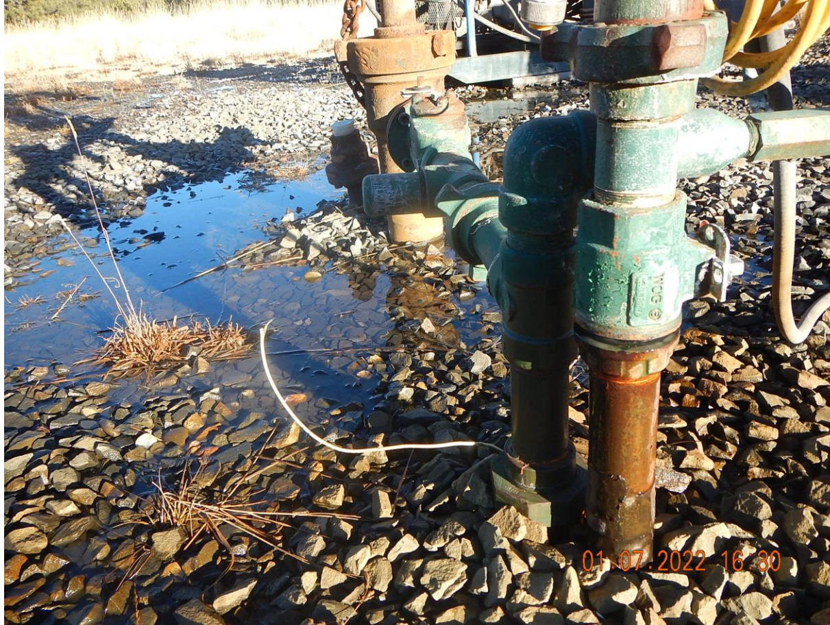
2. Spill source: Broken valve on wellhead waterline
