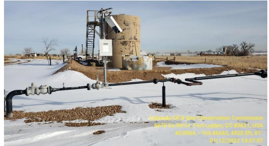
Photo 5 Flow line manifold
