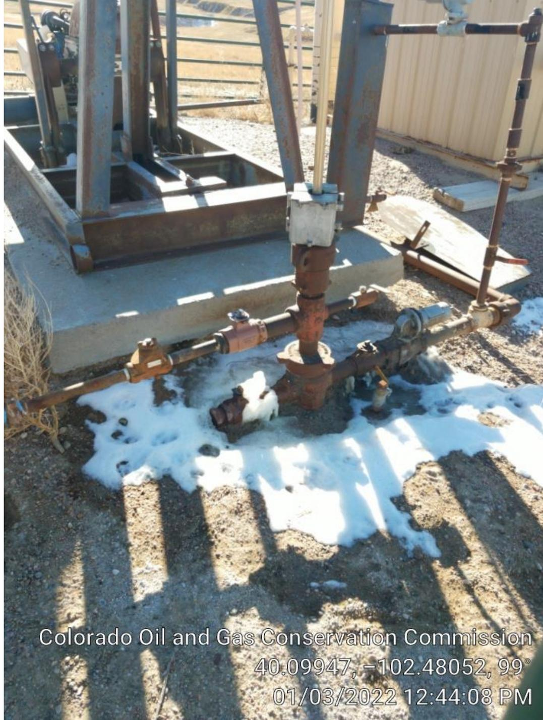
Water valve is dripping as evidenced by the ice forming on the casing below the flowline.
