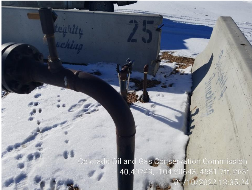
Photo 7 – Unmarked Risers
