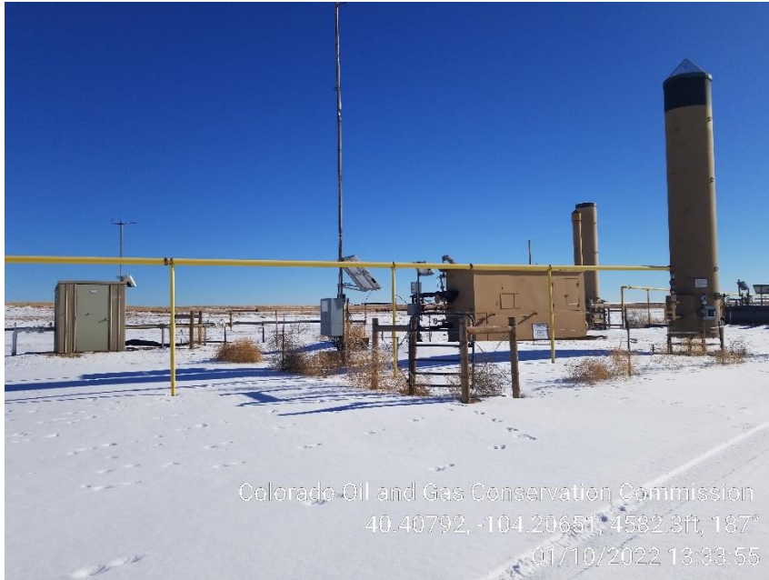
Photo 3 – 41-44-16HZ Separator and ECD
