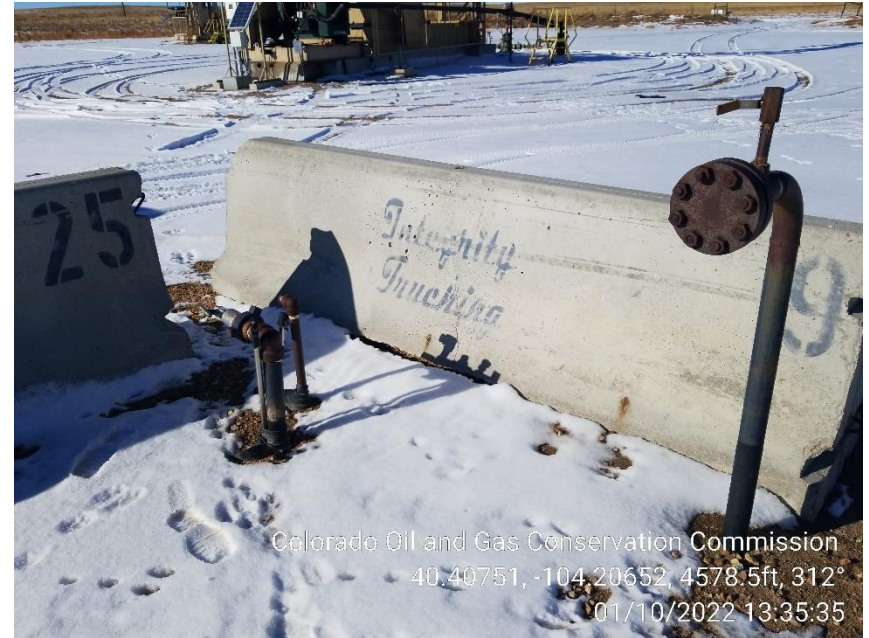
Photo 8 – Unmarked Risers
