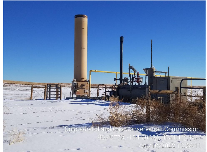
Photo 4 – 31-34-16HNB Separator and ECD
