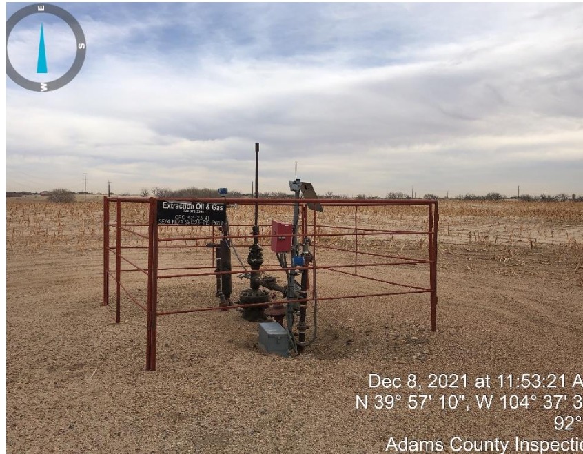
Photo #1 Well Head.
