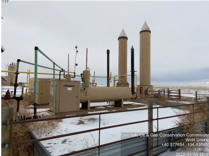
Photo #3 Ball Ranch AC15-65HN Tank Battery / Battery site Inactive / Shut-down ECDs, Separators
