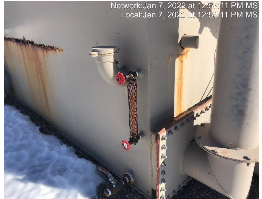
Photo #5628 Sight glass indicates the storage tank is full of an unknown fluid.
