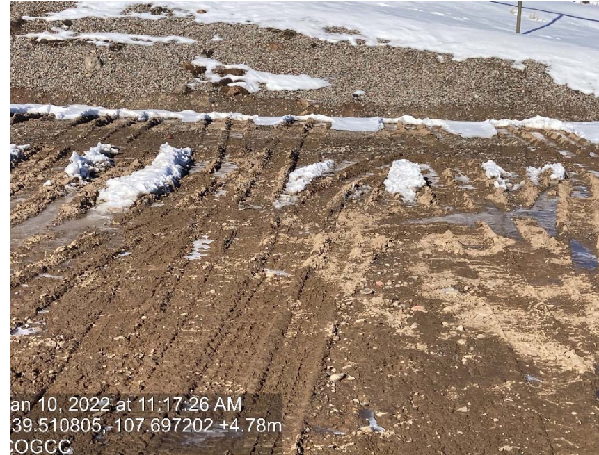
Lack of stabilization/compaction (sight derogation)
