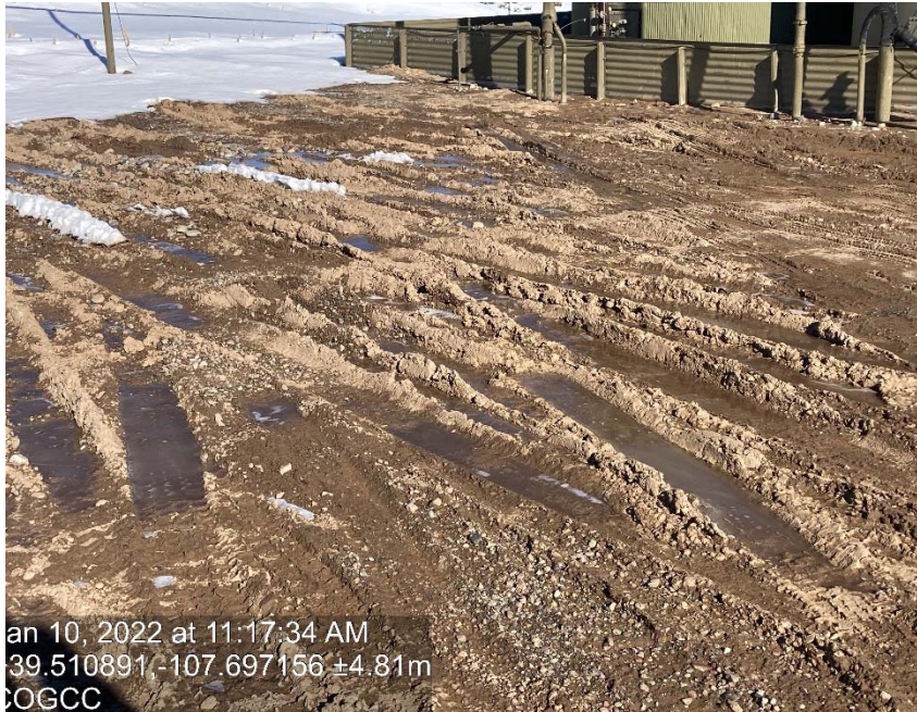
Lack of stabilization/compaction (sight derogation)
