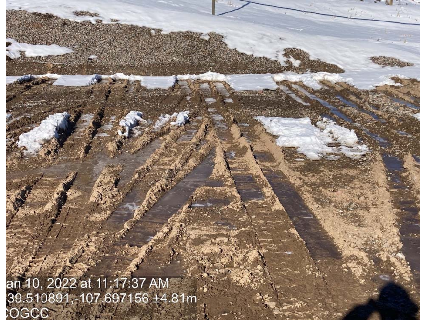
Lack of stabilization/compaction (sight derogation)
