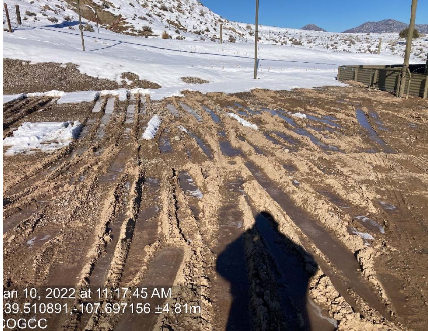
Lack of stabilization/compaction (sight derogation)
