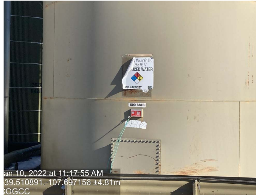
Labeling falling off
