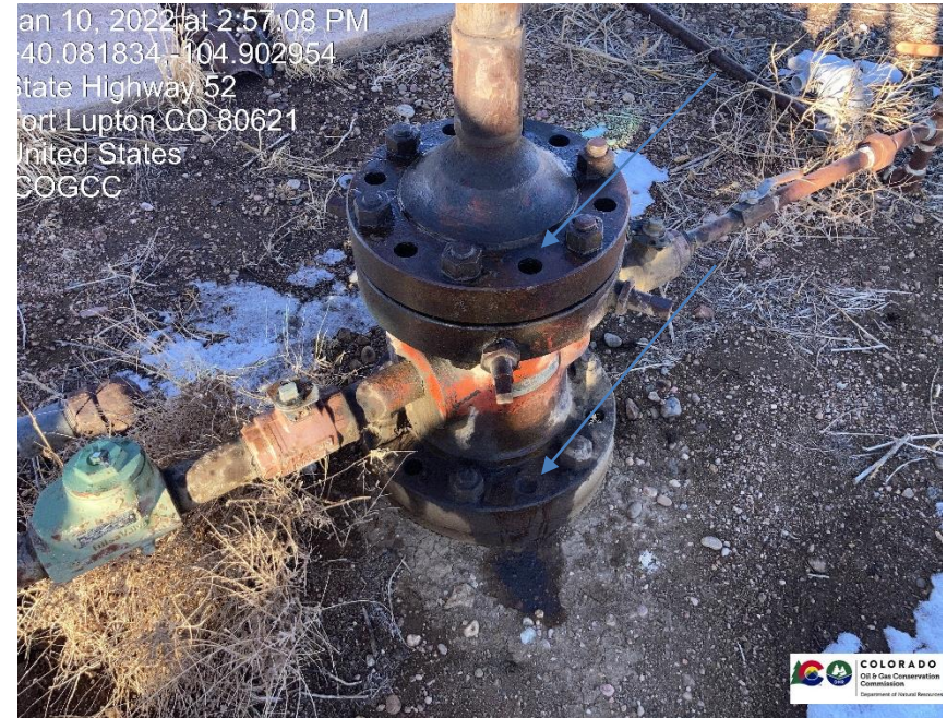
Pic 2 wellhead. Wellhead bolts are missing on both tubing, and production casing hanger. Mechanical integrity issue are visible due to leaking wellhead on flanged connections.
