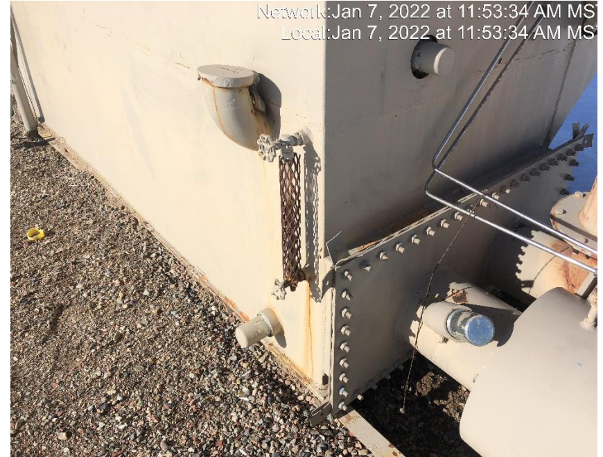
Photo #5624 Sight glass indicates the storage tank is full of an unknown fluid.
