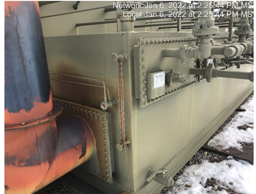
Photo #5619 Sight glass indicates the storage tank is full of an unknown fluid.
