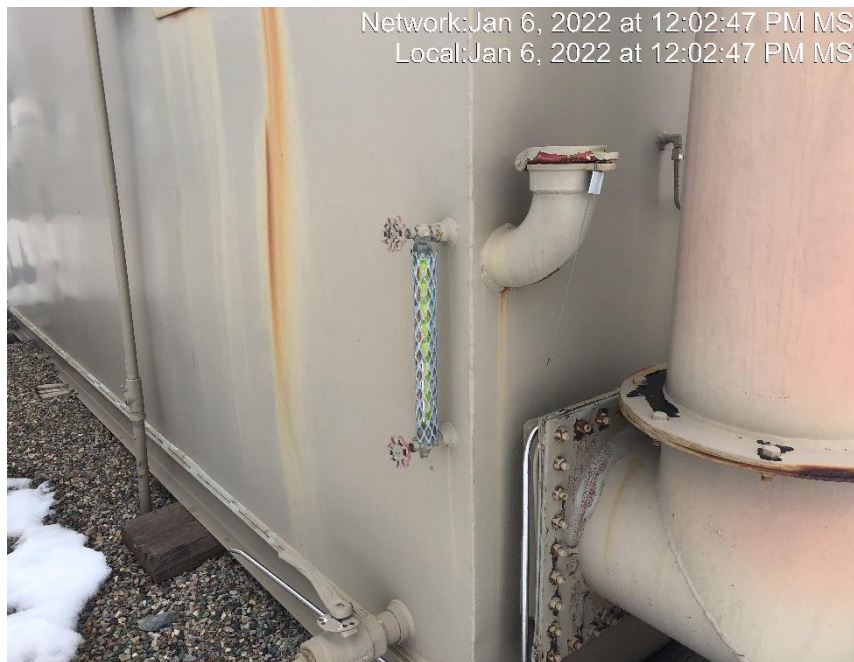
Photo #5601 Sight glass indicates the storage tank is full of an unknown fluid.
