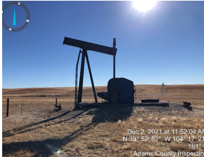
Photo #1 Pump Jack.
