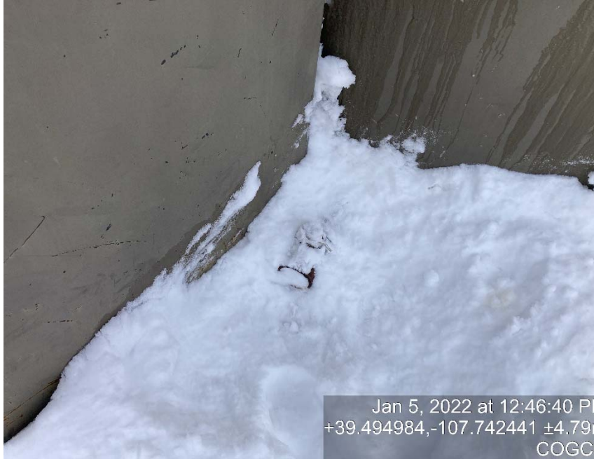
Load lines lacking bull plugs/caps
