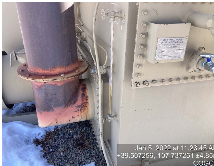
Storage tank sight glass shows fluid
