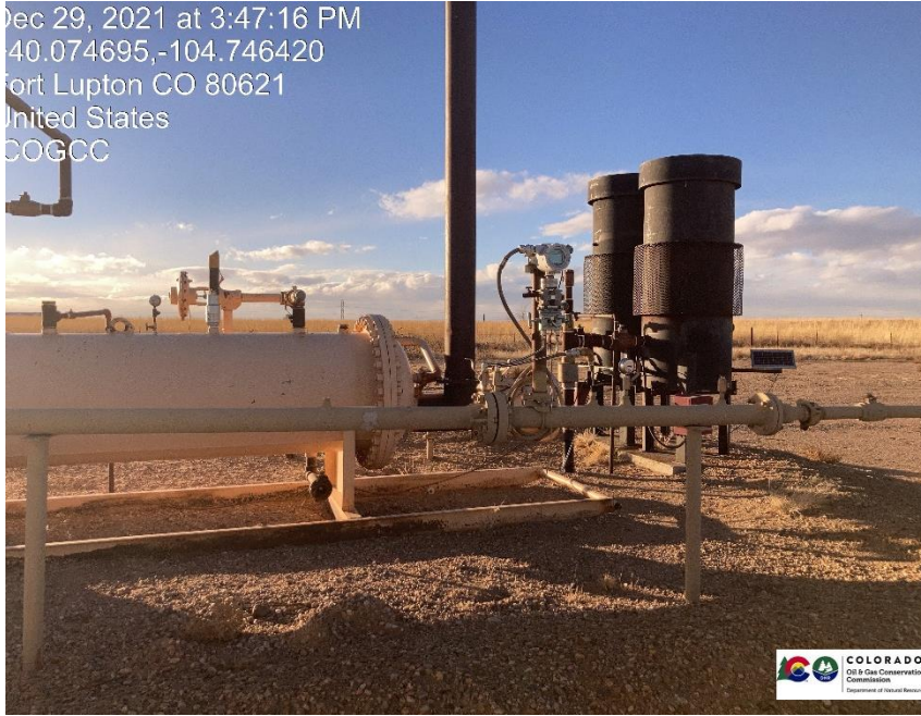
Pic 3 gas meter run appears to have been replaced with digital gauge not active at time of inspection.
