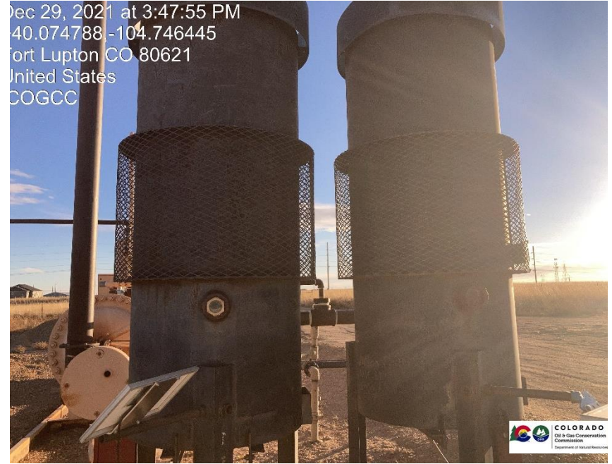
Pic 4 2 ECD on location appear to be burning gas constant.
