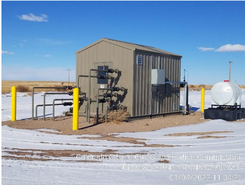
Photo 3 – Gas Lift Injection Meter House
