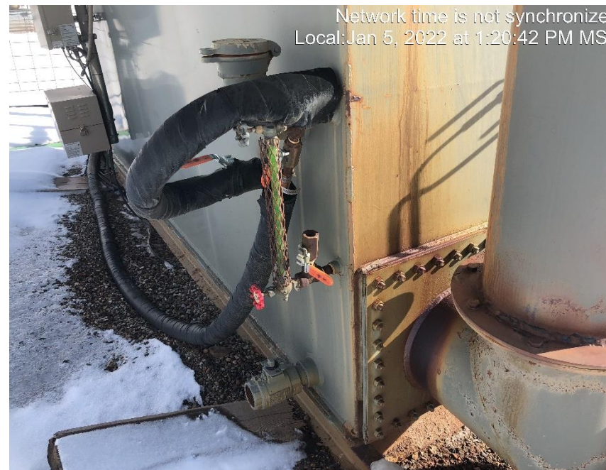
Photo #5593 Sight glass indicates the storage tank is full of an unknown fluid.
