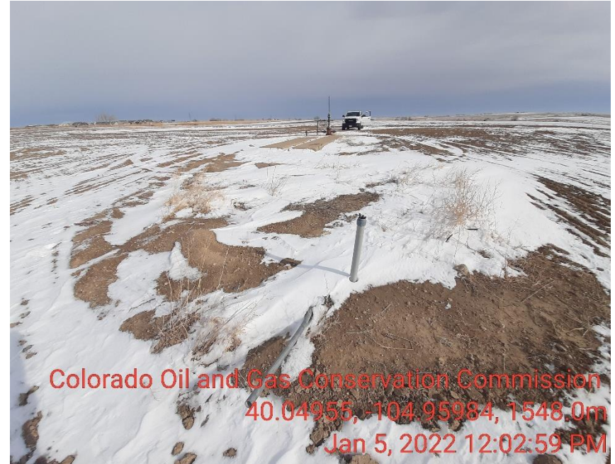
Photo 2 Unmarked electric riser.
