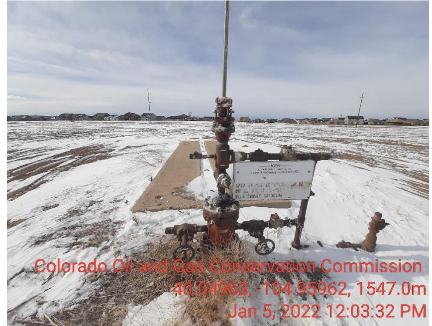
Photo 4 No Braden head visible.
