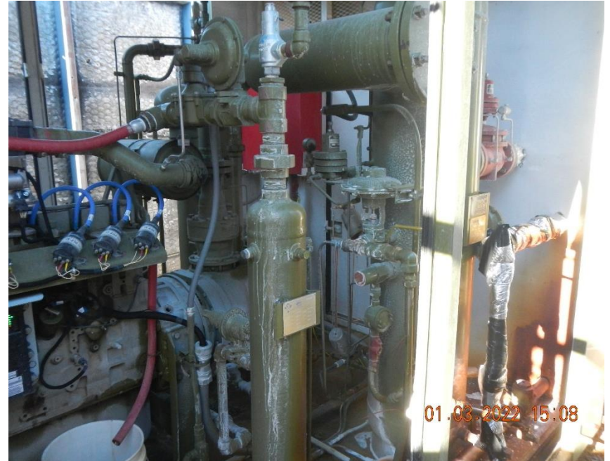
Equipment on compressor skid is stained with white residue.
