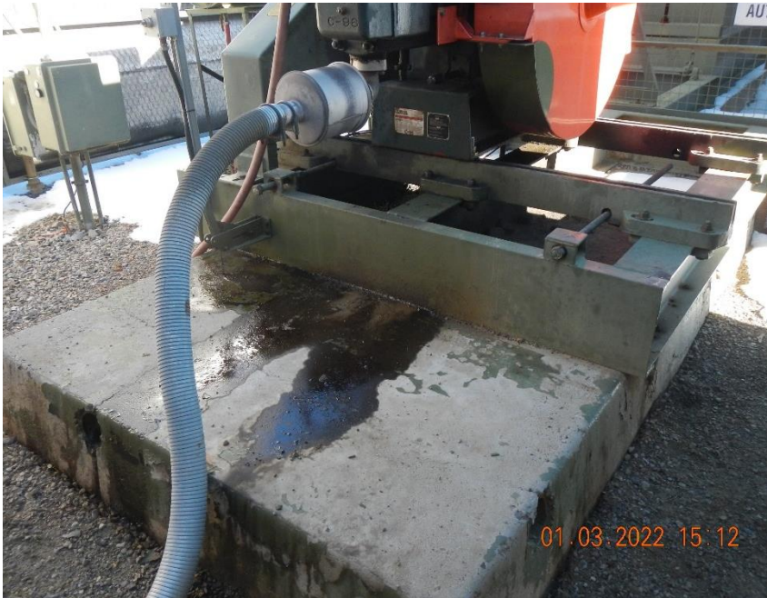
Concrete pad is stained and wet beneath prime mover.
