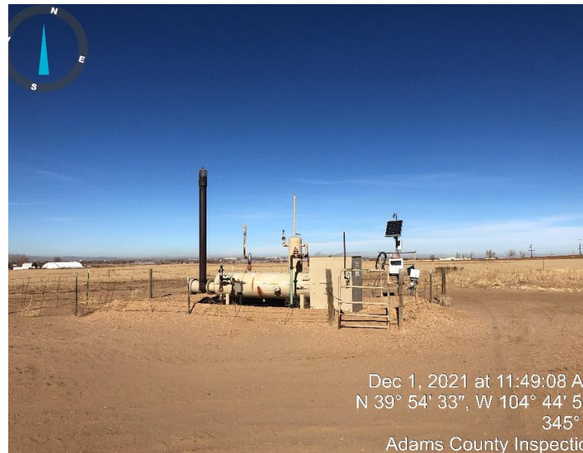
Photo #2 Meter & Separator.
