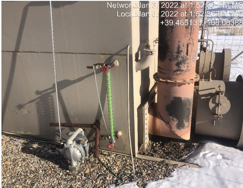
Photo #5562 Sight glass indicates the storage tank is full of an unknown fluid.
