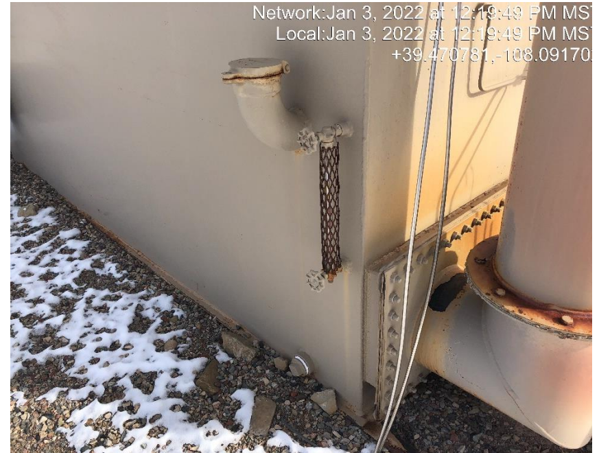
Photo #5552 Sight glass indicates the storage tank is full of an unknown fluid.
