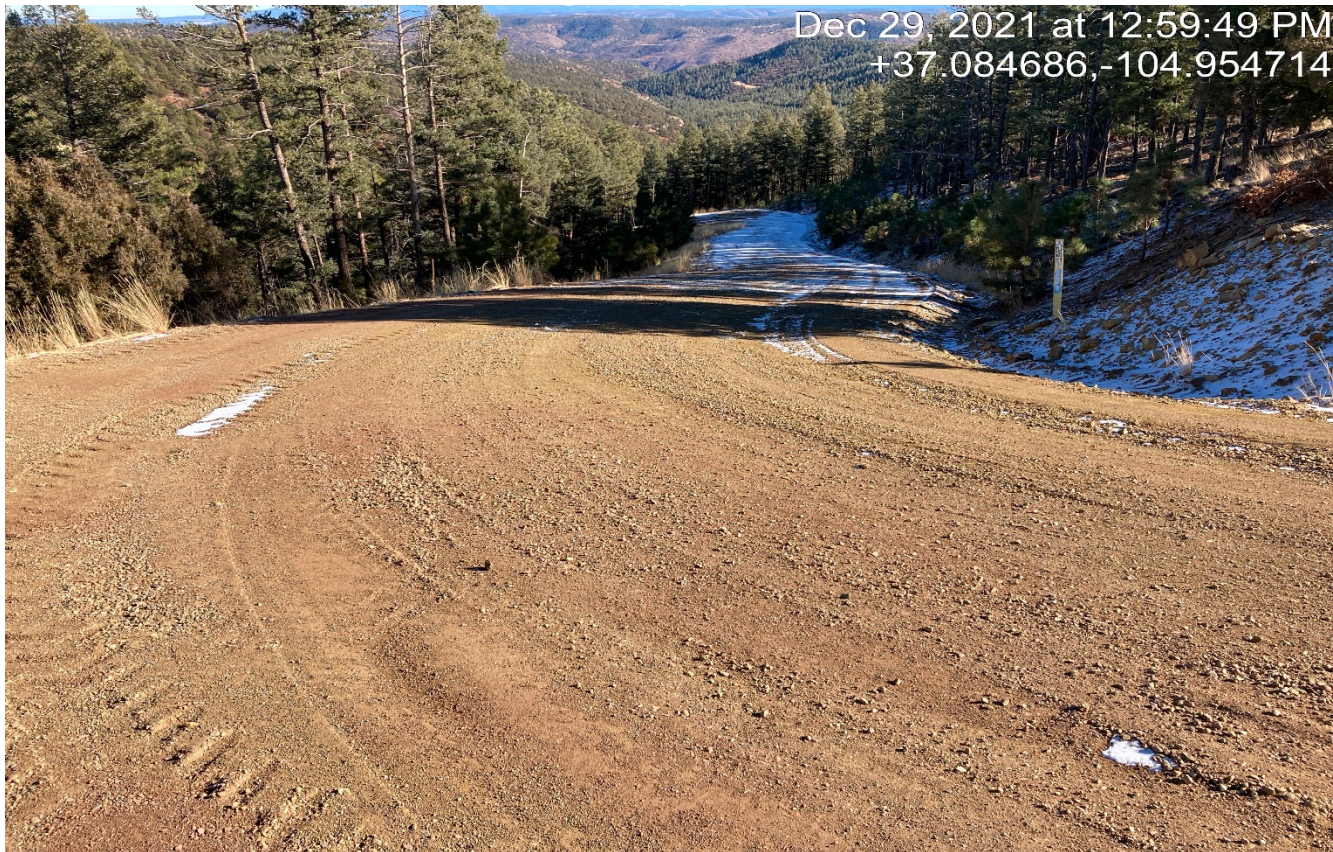
Photo 1. Facing east along the access road. The road has been regraded.
