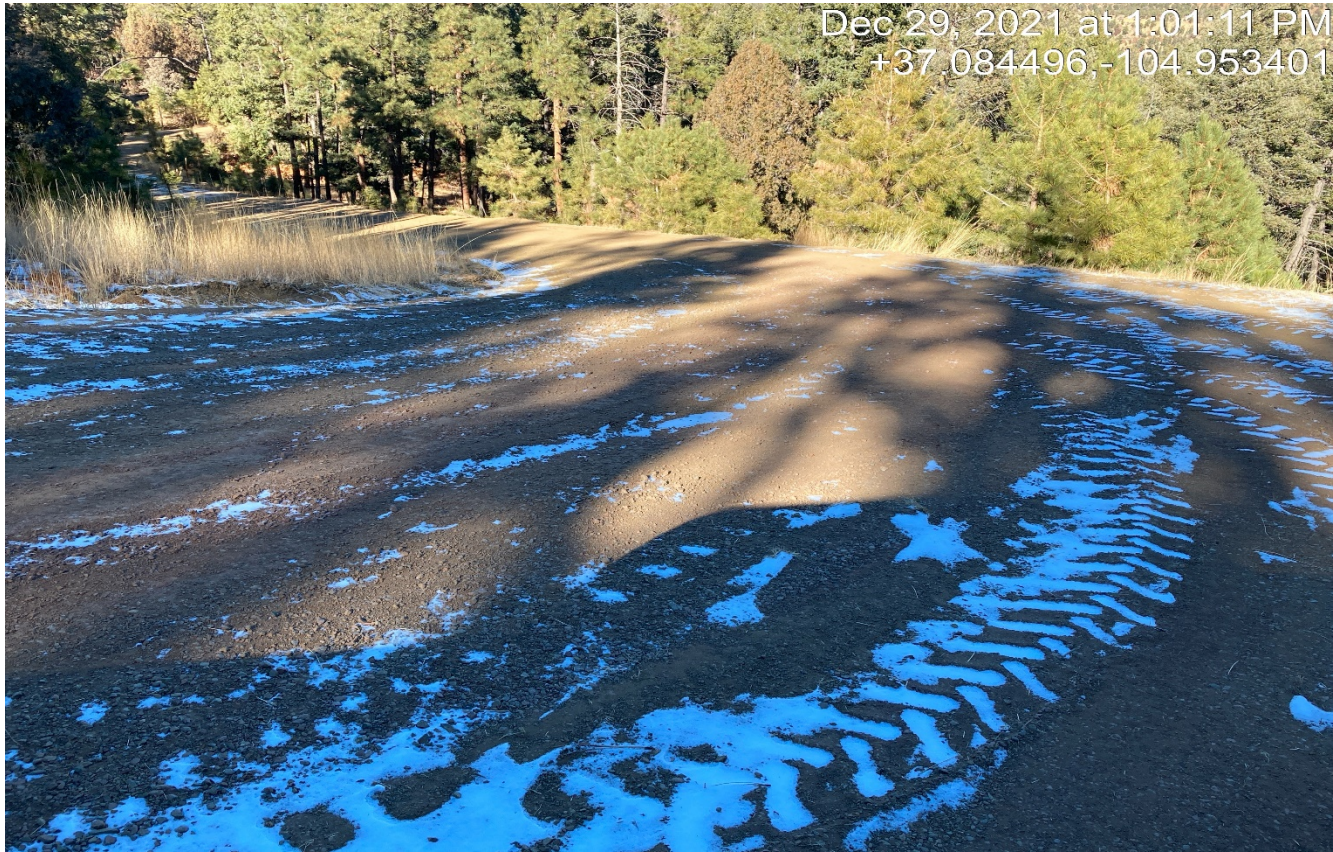
Photo 2. Facing northwest along the access road. The road has been regraded.
