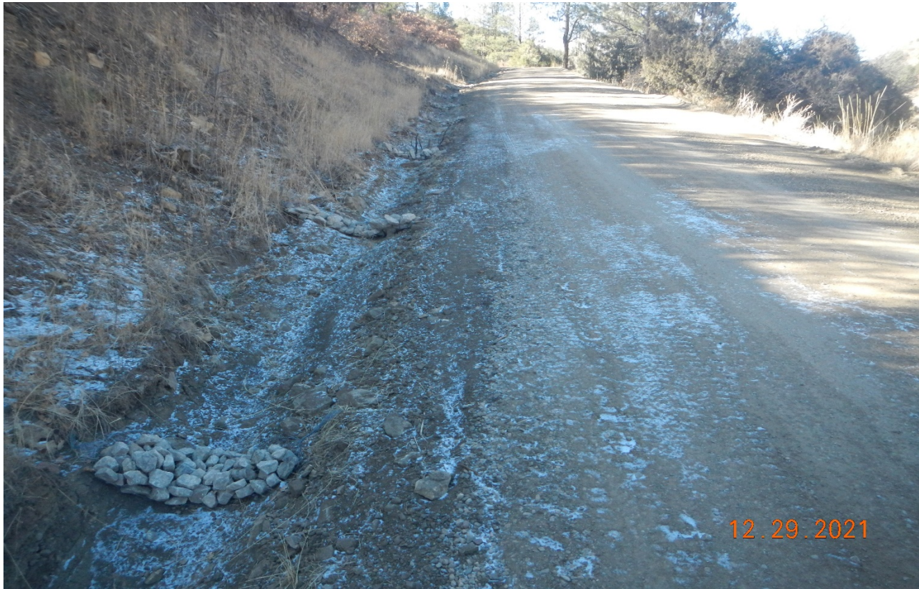
Photo 2. BMP's have been installed along the steep portion of the road to prevent erosion but will require ongoing maintenance.
