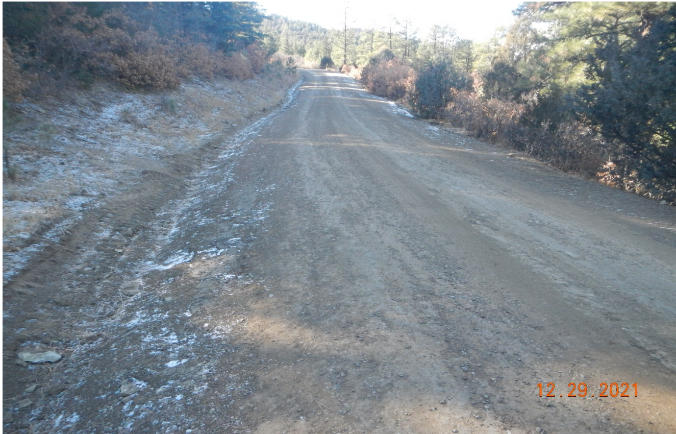
Photo 3. The road has been regraded and culverts are now maintained.
