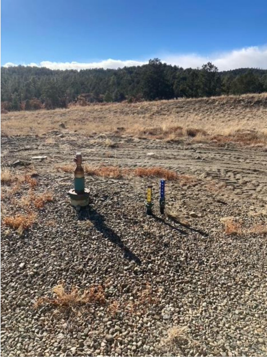
Labeled and LO/TO unused risers to comply with Rule 606
