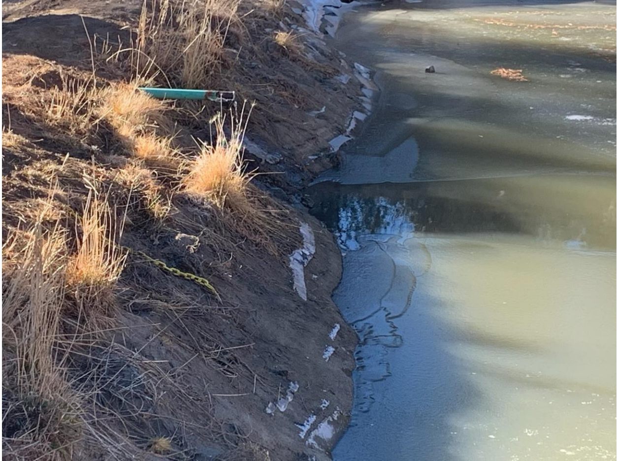
Lowered fluid level so at least two feet of freeboard exist per Rule 909.c.
