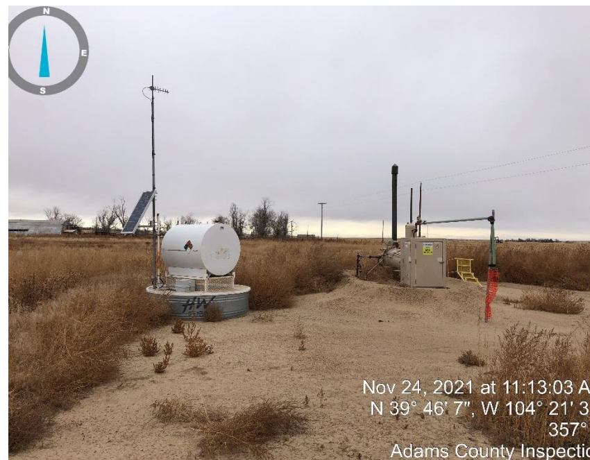
Photo #2 Separator and chemical tank.
