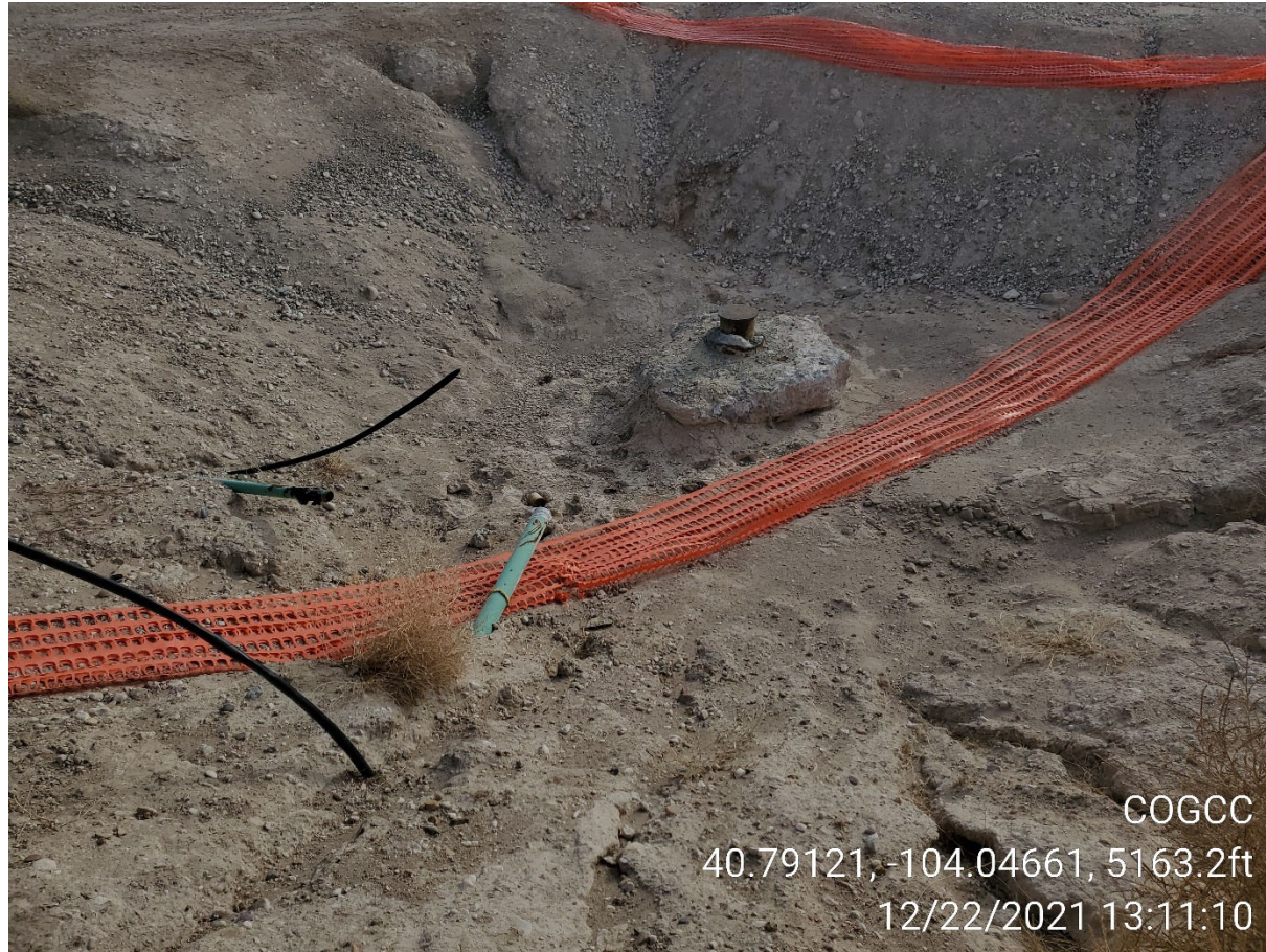
Photo 3 Open excavation at well with flowline exposed
