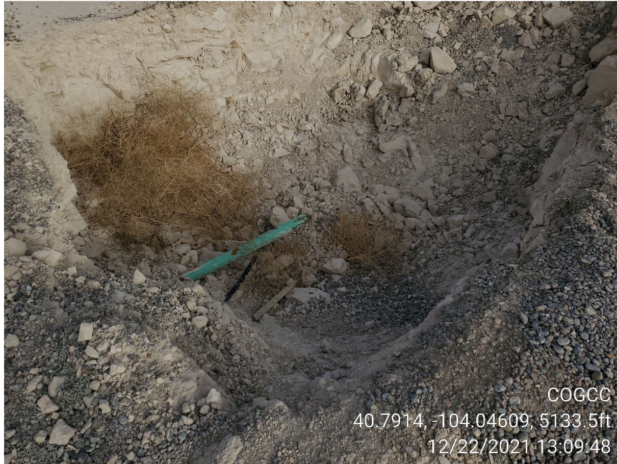
Photo 1 Open excavation with flowline exposed
