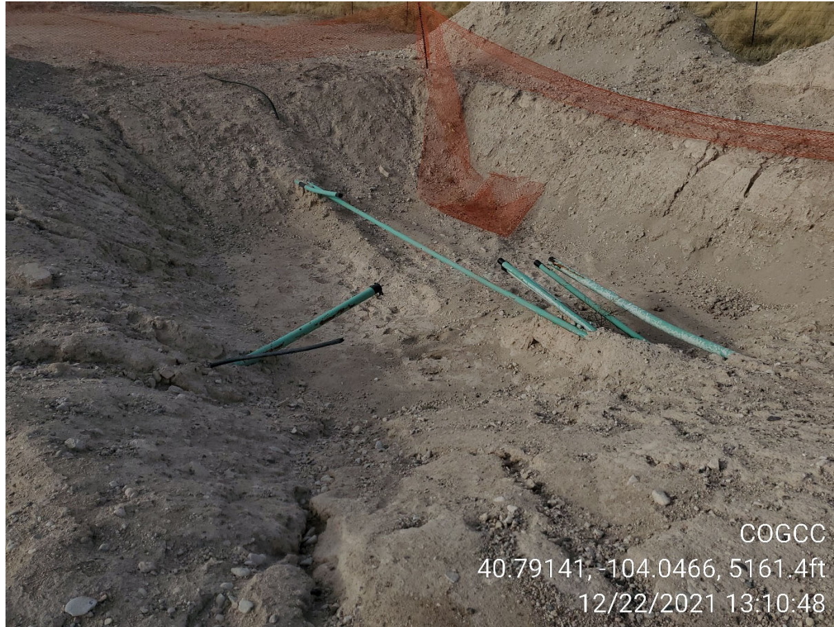
Photo 2 Open excavation with flowline and dump lines exposed
