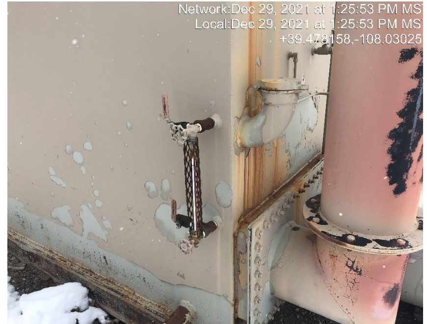
Photo #5538 Sight glass indicates the storage tank is full of an unknown fluid.
