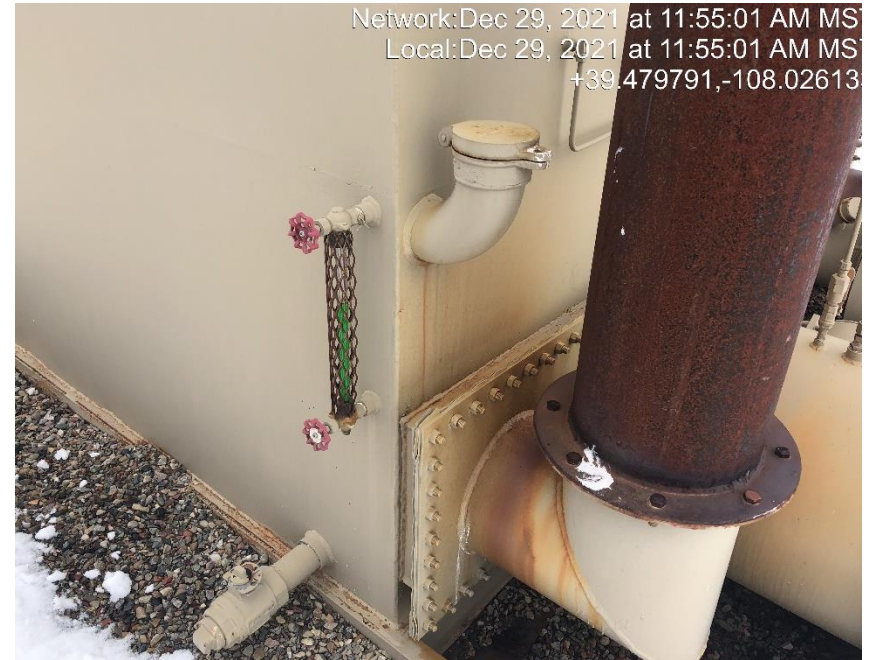
Photo #5531 Sight glass indicates the storage tank is full of an unknown fluid.
