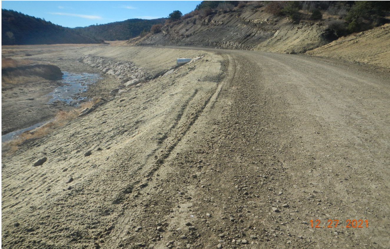
Photo 2. The side of the main road and stream bank has been resloped and stabilized.
