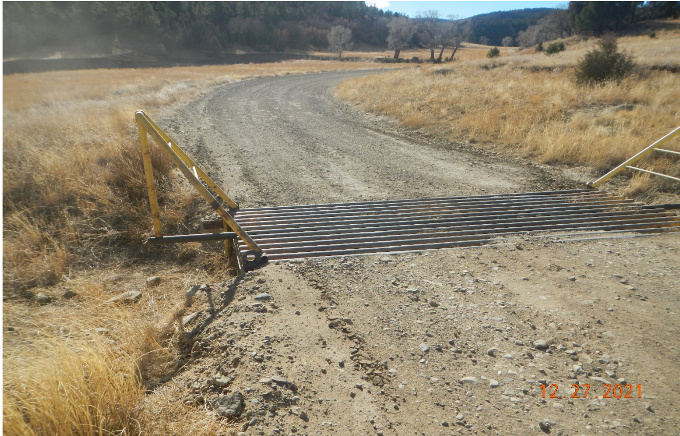
Photo 5. The cattle guard along the road has been repaired.
