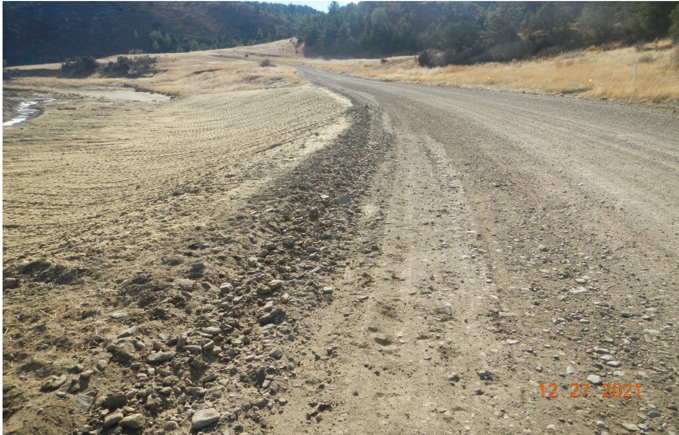
Photo 4. The side of the main road and stream bank has been resloped and stabilized.
