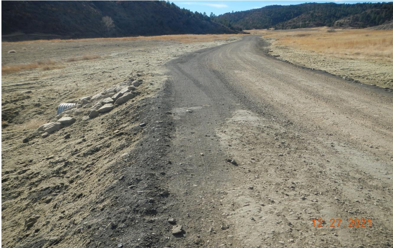
**Photo 3.** The area of erosion further along the road has been repaired and a culvert has been installed.
