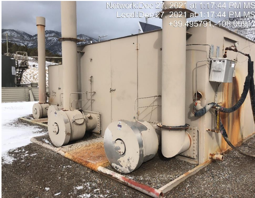
Photo #5515 Storage tank not legible.
