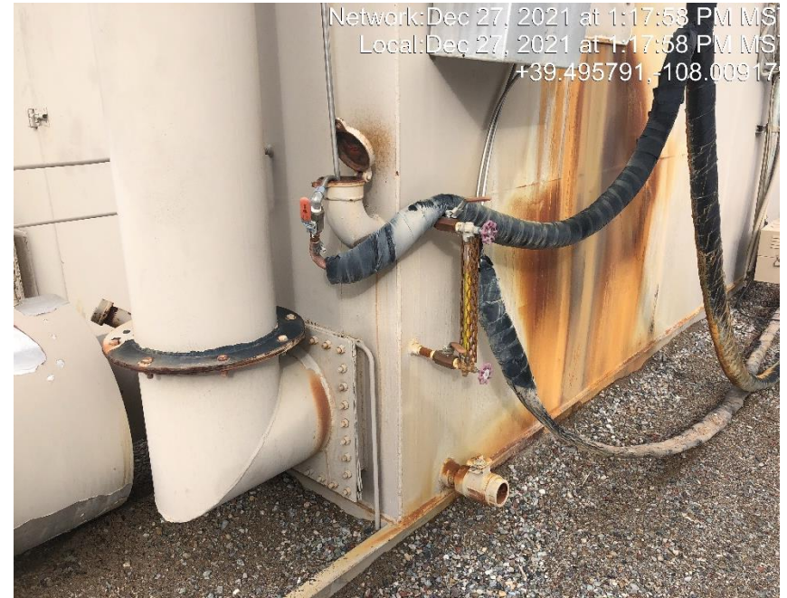
Photo #5516 Sight glass indicates the storage tank is full of an unknown fluid.
