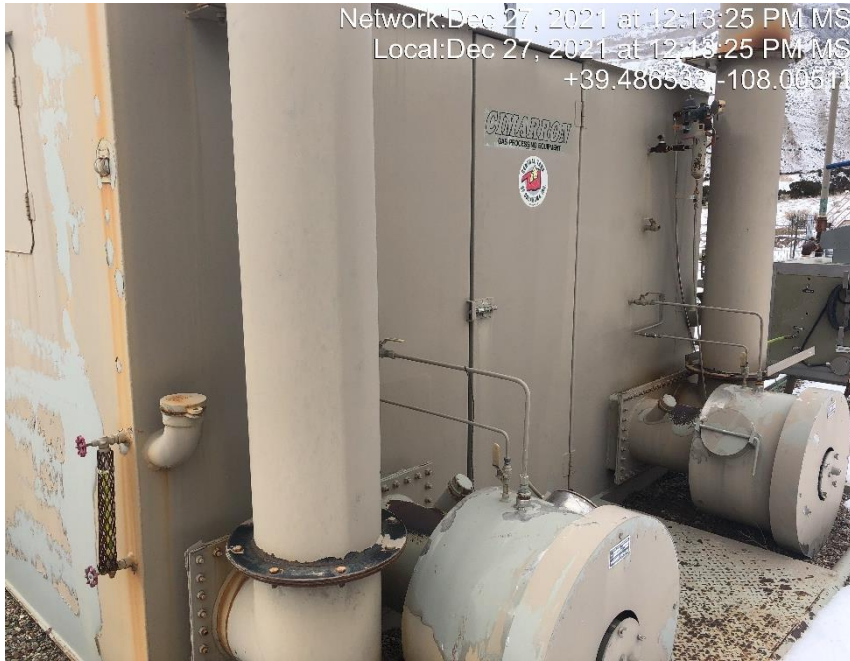
Photo #5505 Storage tanks not labeled.
