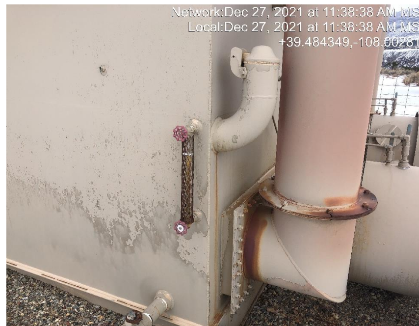
Photo #5502 Sight glass indicates the storage tank is full of an unknown fluid.
