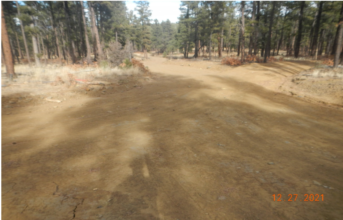
Photo 1. Facing north toward the access road. There is a berm and runoff ditch in this area of the road. The road has been regraded.
