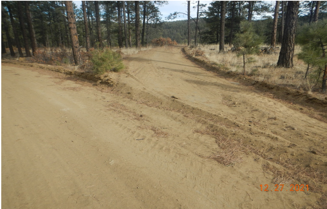
Photo 2. There are stormwater ditches carved away from the road. The disturbed loose soils are susceptible to erosion and need to be seeded and stabilized where the ditch disturbance has occurred.
