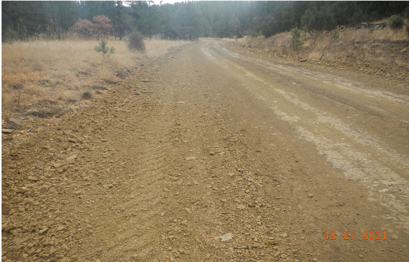
Photo 1. Facing southeast along the road. Areas of erosion along the road side have been filled in and repaired.
