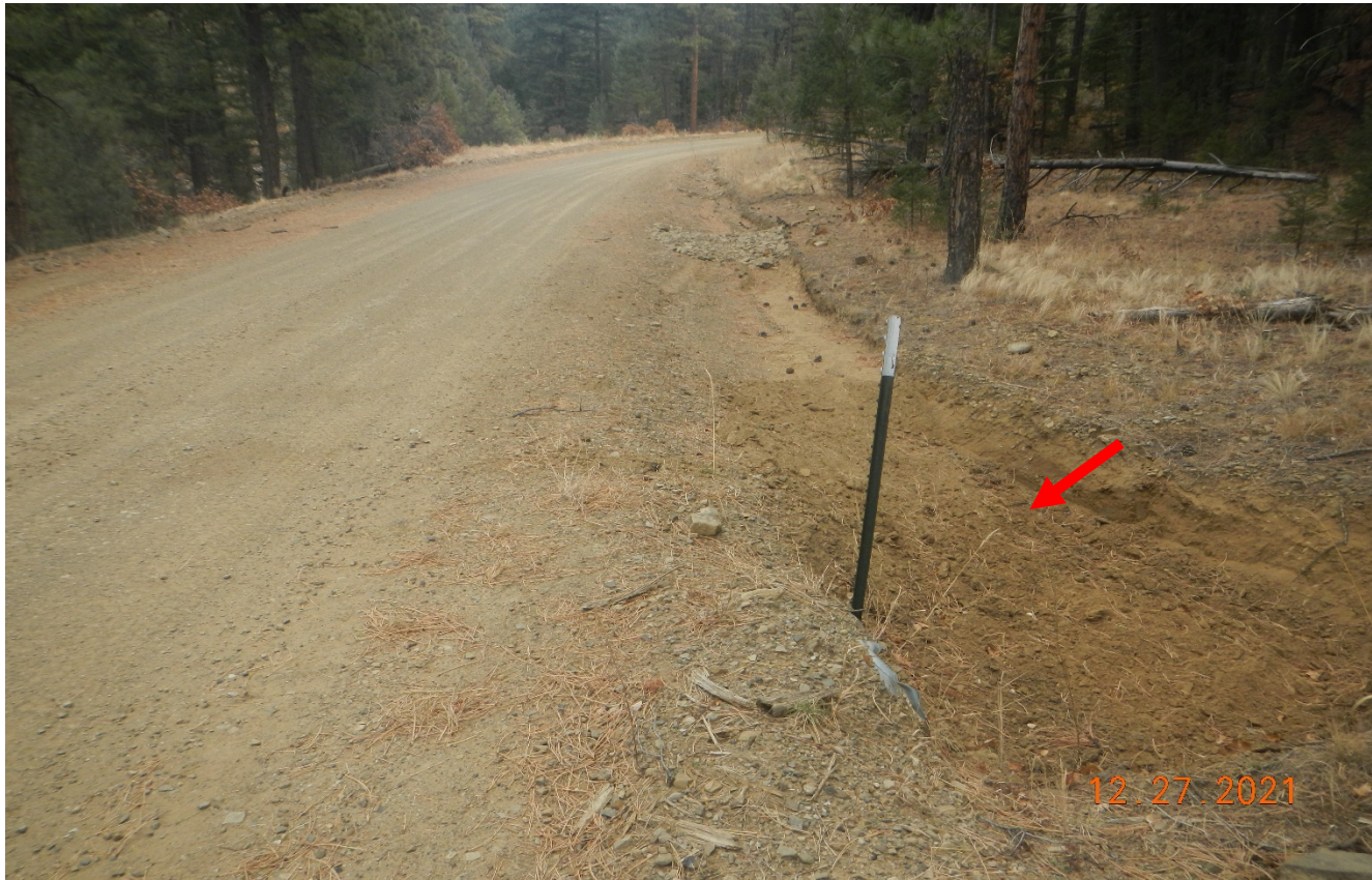
Photo 3. The culverts along the road have been cleaned out and maintained.
