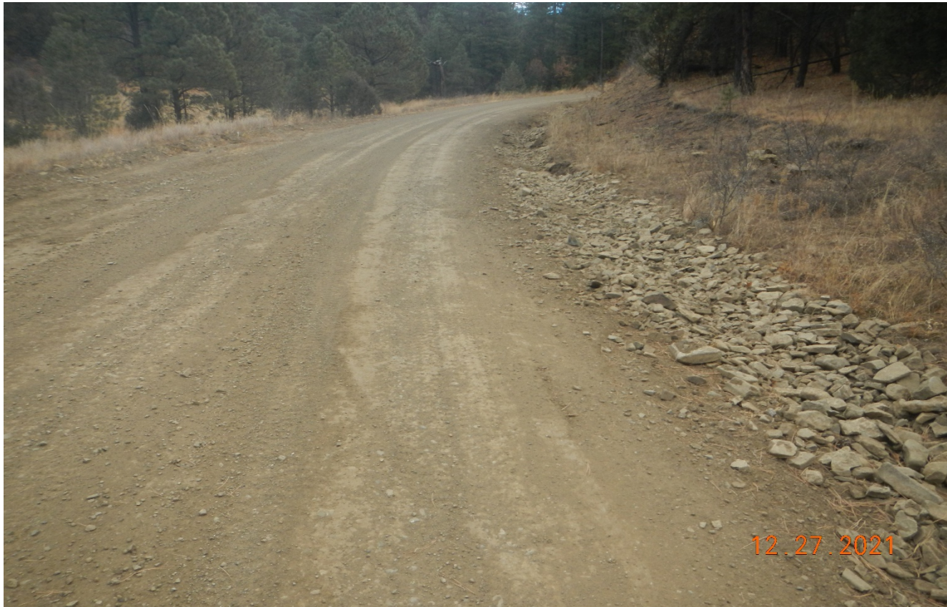
Photo 2. Facing southeast along the road. Areas of erosion along the road side have been filled in with rock rip/rap.
