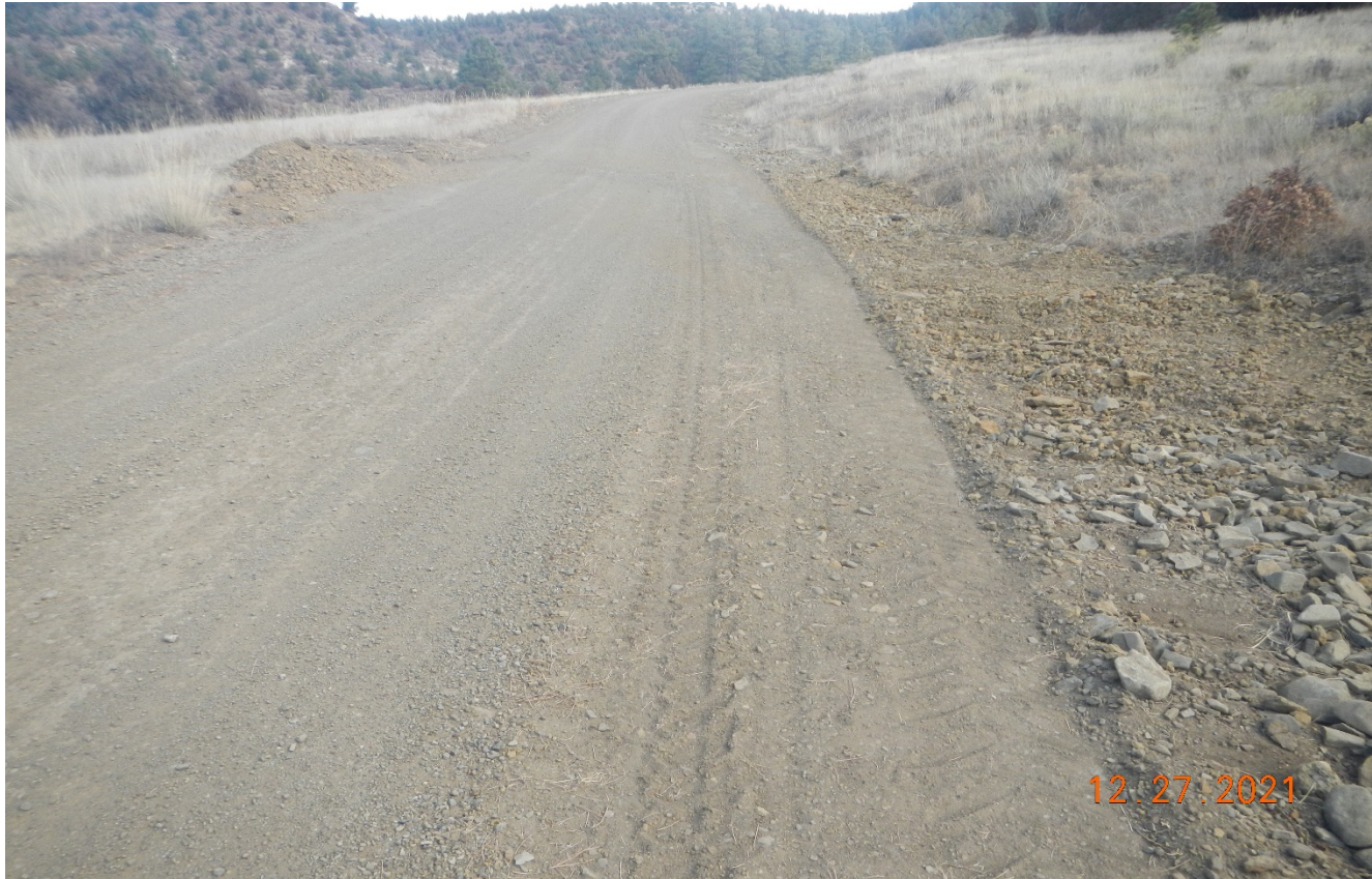
Photo 4. Facing northeast along the road. Areas of erosion along the road side have been filled in and repaired.
