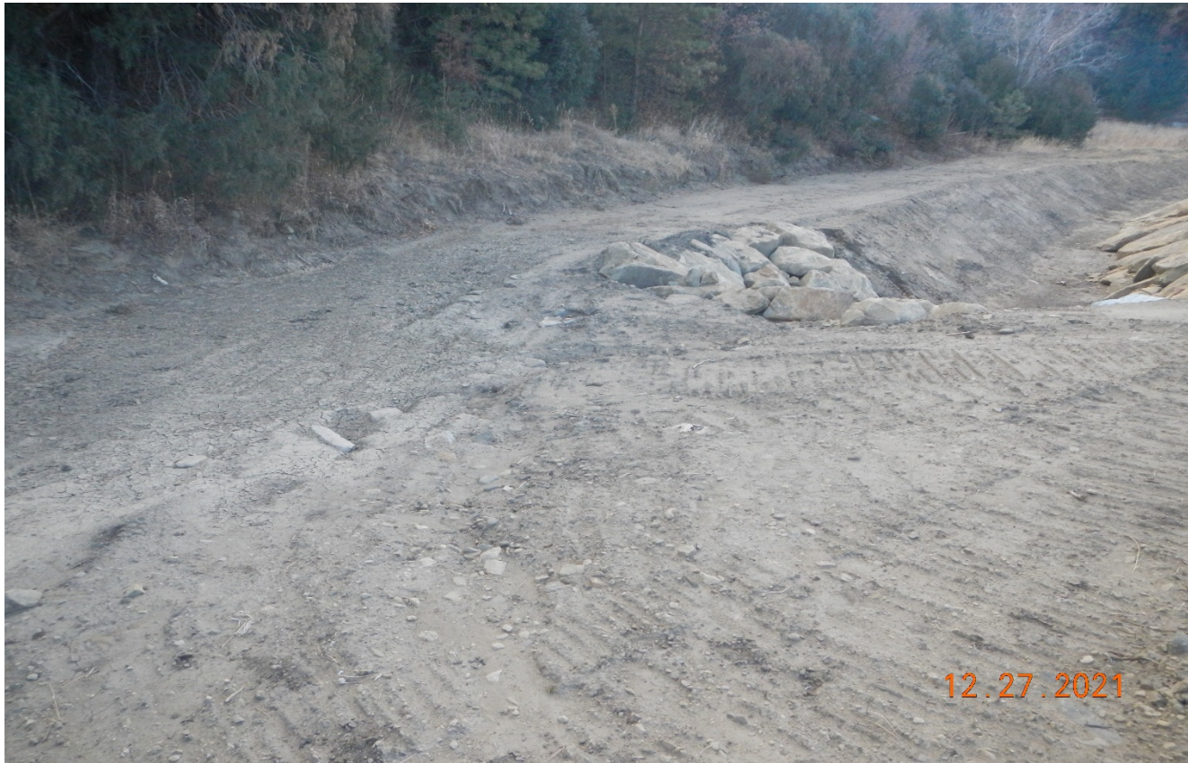
Photo 3. Facing at south side of the road at the additional culvert inlet. Disturbed bare soils have not been seeded and stabilized.
