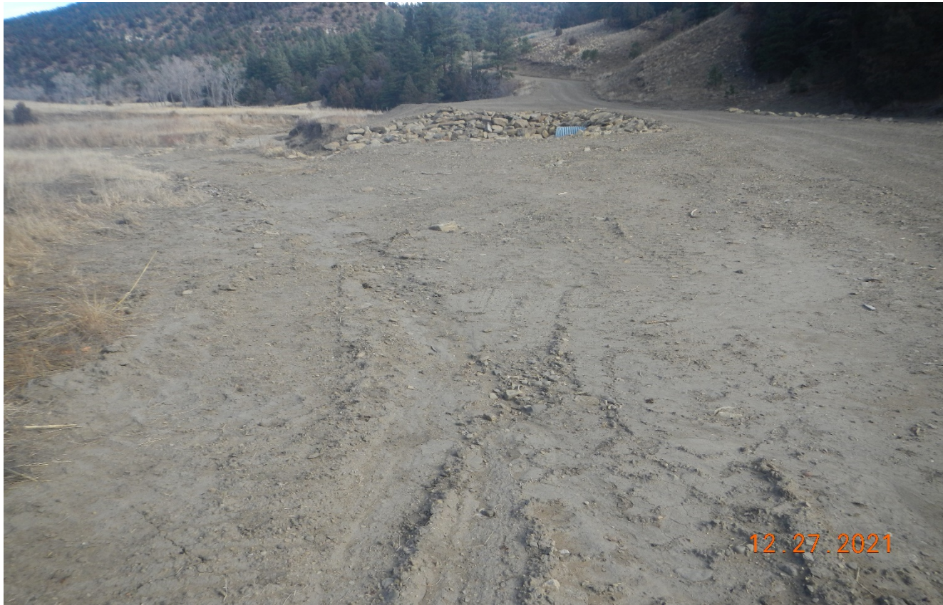
Photo 1. The disturbed bare soils along the roadside at the creek crossing have not been seeded and stabilized. Previous corrective action was not completed.
