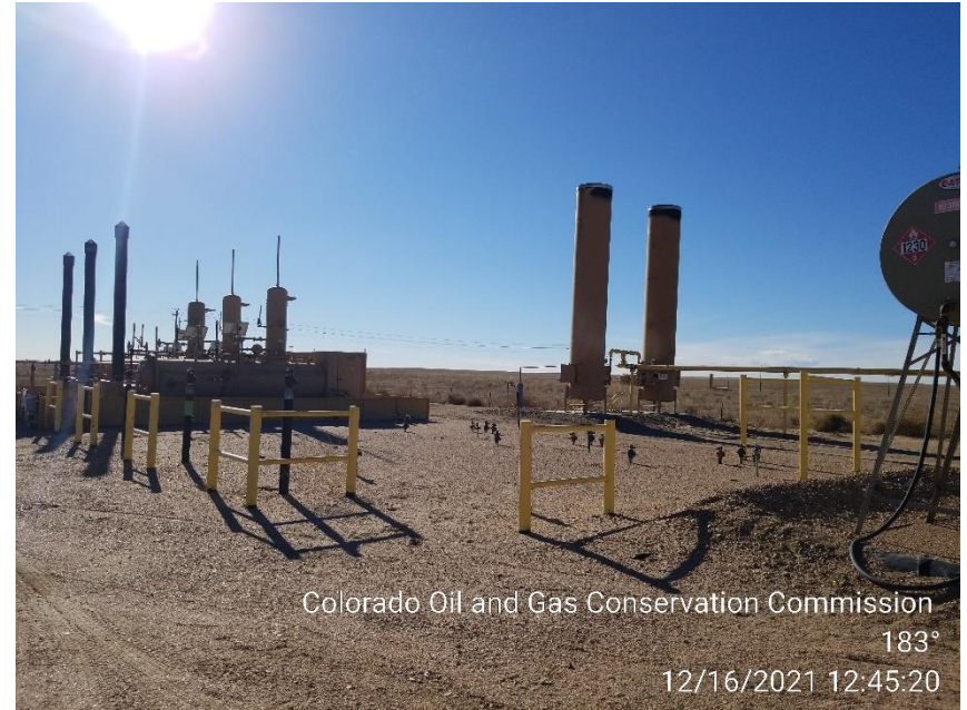
Photo 6 – Separators and ECDs
