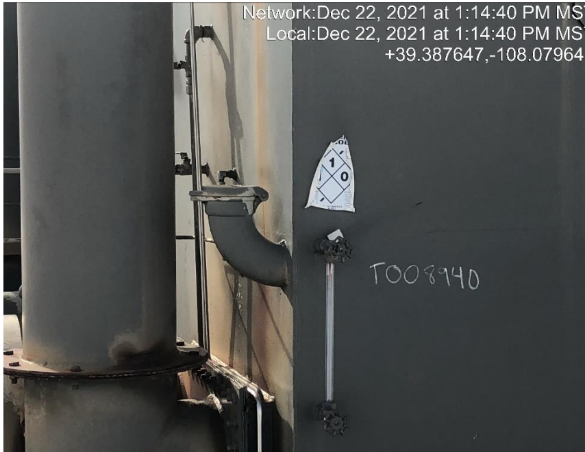
Photo #5490 Separator bath labels weathered and not legible.
