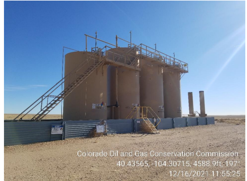
Photo 4 – Tank Battery
