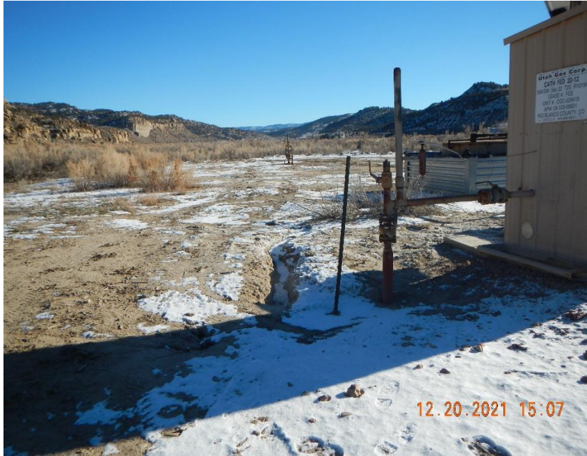
Rilling and channeling by the meter shed.
