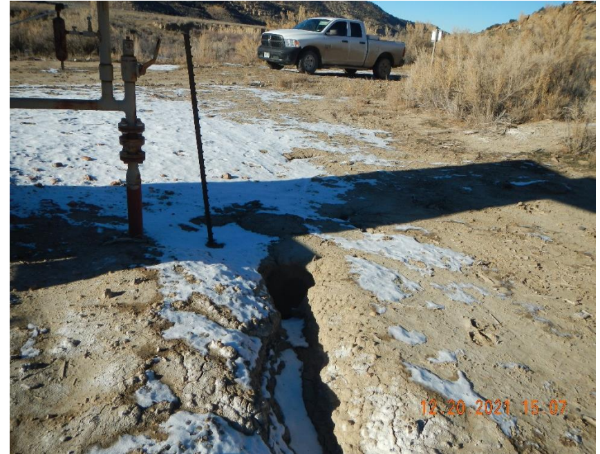
Rilling and channeling by the meter shed.
