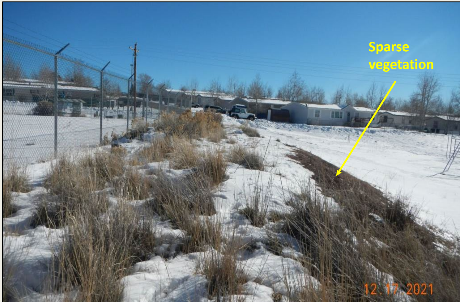
Photo 2. View of the southern project area from the southwestern corner facing eastward. Revegetation is progressing with crested wheatgrass, intermediate wheatgrass, and smooth brome. Sparse vegetation on the southern fill slope needs to be assessed during the 2022 growing season and determine whether spot seeding is needed.
